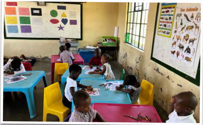
Classroom in disrepair
