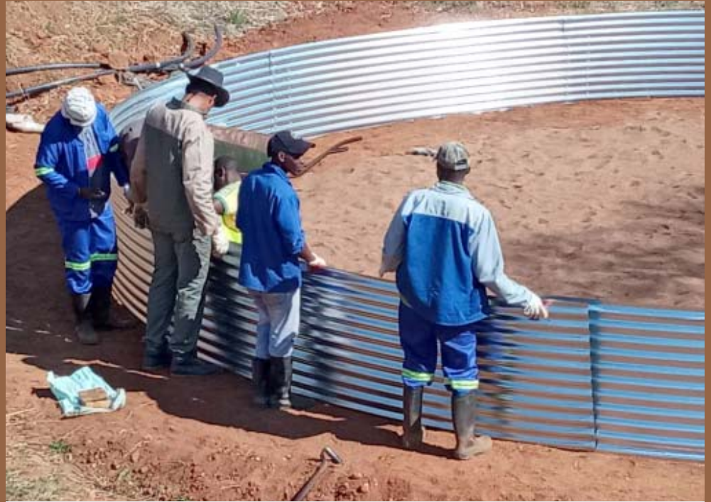
Building the Irrigation System
